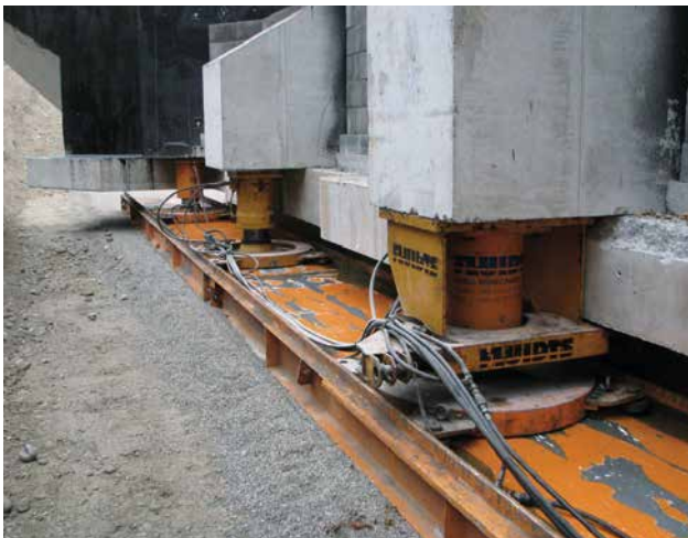
above: "Pushing" Launching on HEB girders and height-adjustable launching bearings
