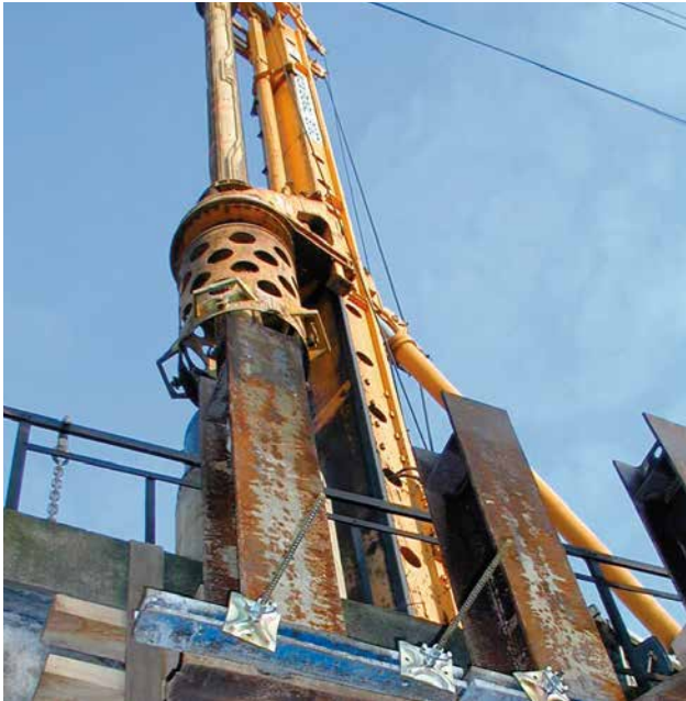
Railway bridge Siemensstraße in Frankfurt Construction of bored piles in track area
