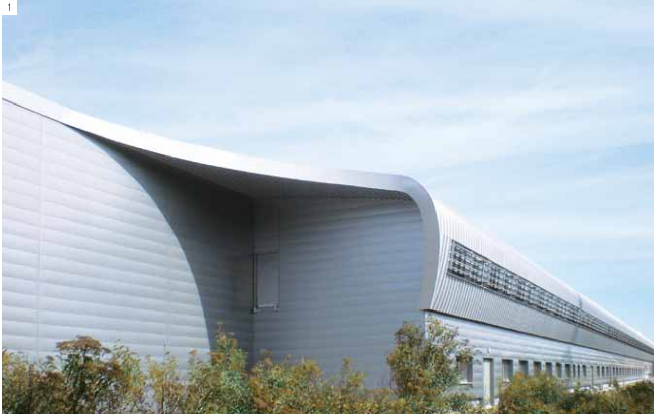
1 Transition train hall to operation building at line 6 2 Canopy geometry roof skin made of profiled metal sheets
