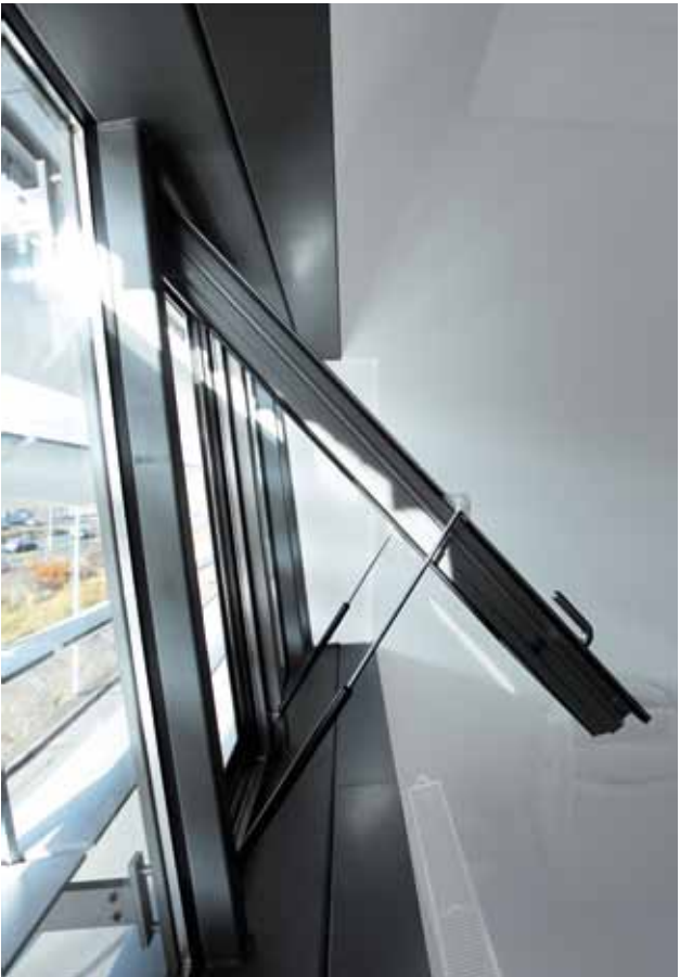
Top-hung window in inclined post/bar façade
