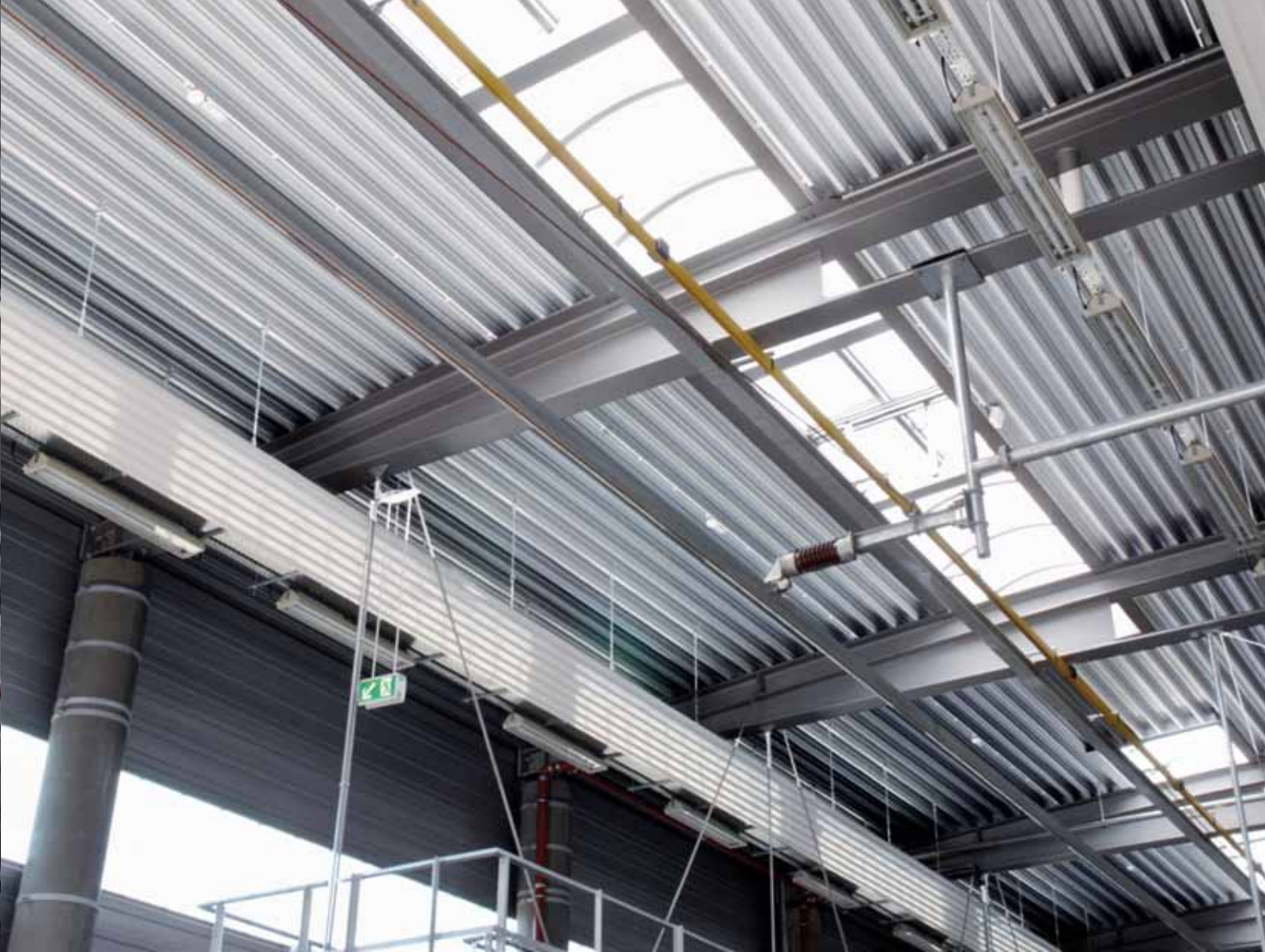
Roof truss with suspended working platforms and train energy supply
