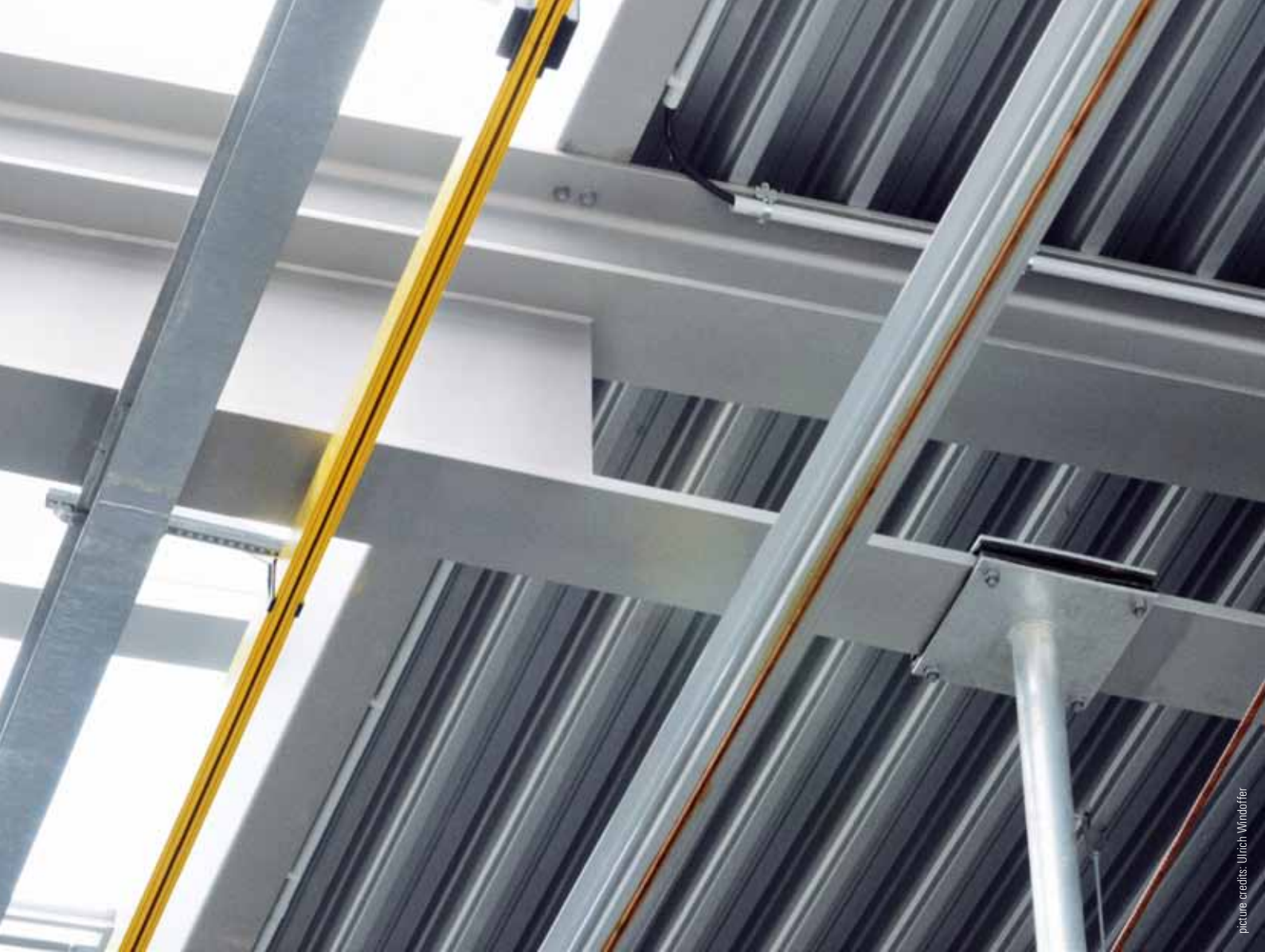
Detail of roof truss connected roof girders
