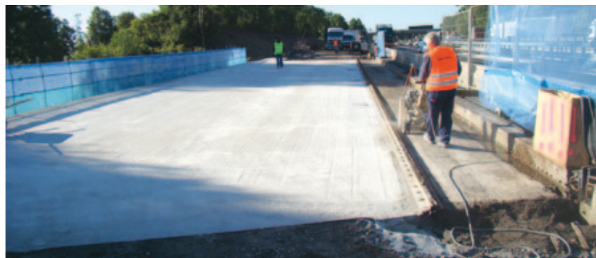
Fig.7, Demolition of asphalt, caps and sealing
