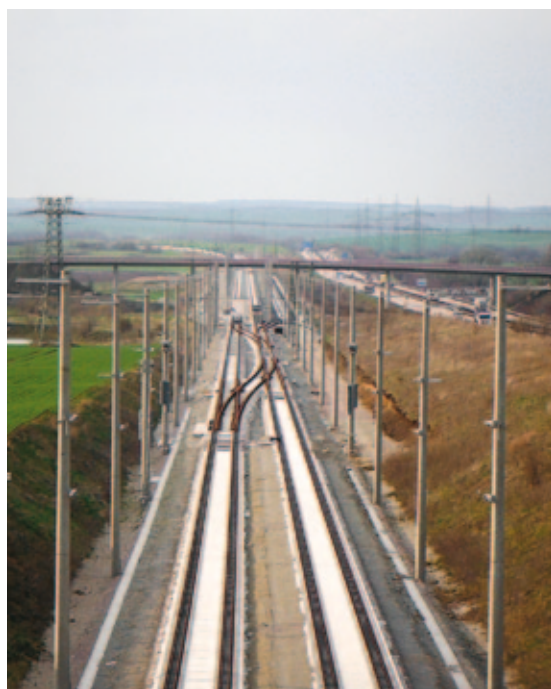
Fig.5, Ballastless track Ilmenau – Erfurt, switch connections during construction; crossovers; in the background one of two overtaking stations, track structure station in ballasted track
