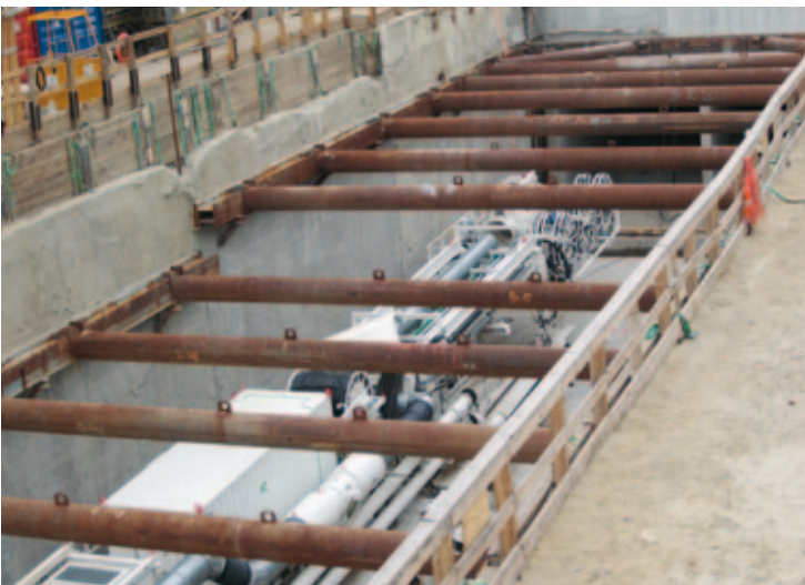
Fig.6, TBM under stiffened TSS
