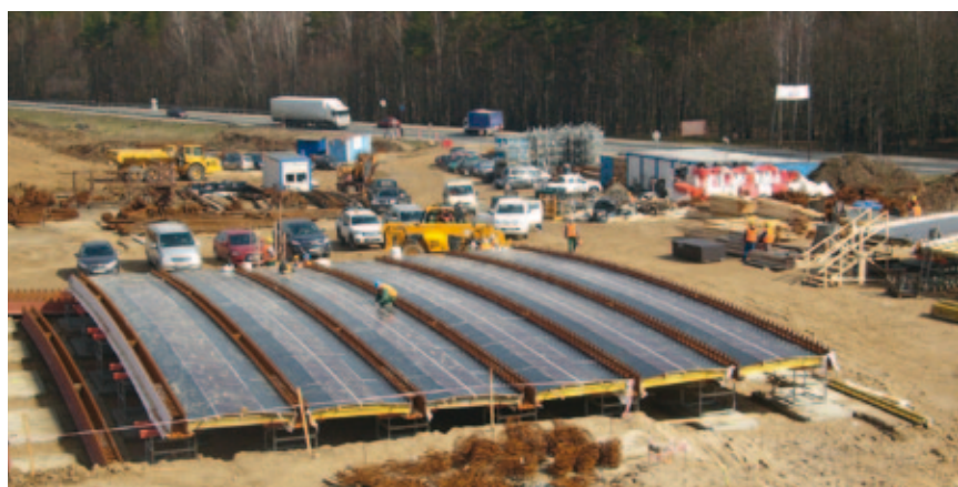
Fig.3, Fabrication area for concreting of prefabricated elements directly next to the construction site
