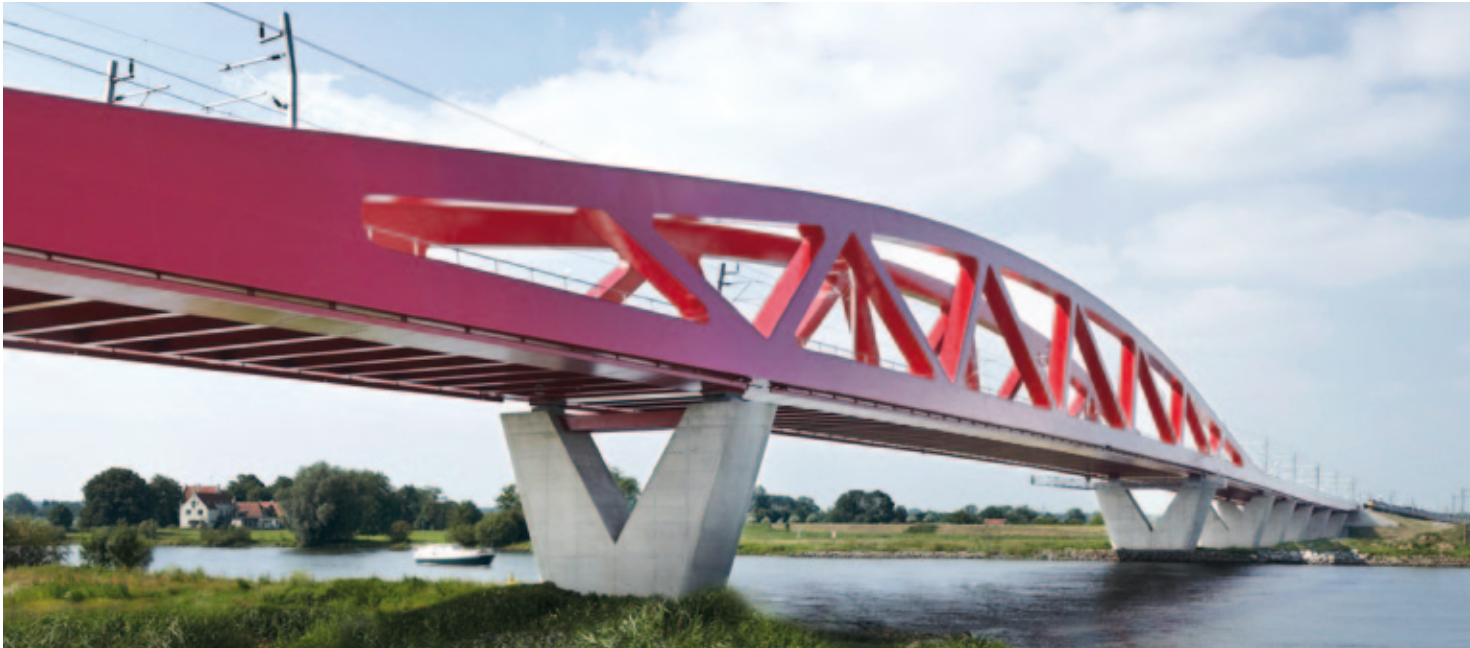
Fig.2, Bridge over the IJssel, view on the main opening over the River IJssel with a span width of 150 m; total bridge length approx. 926 m
