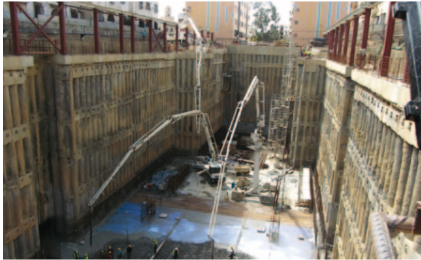
Fig. 12, Terminus Ain Naadja 2 area west, concreting of floor slab
