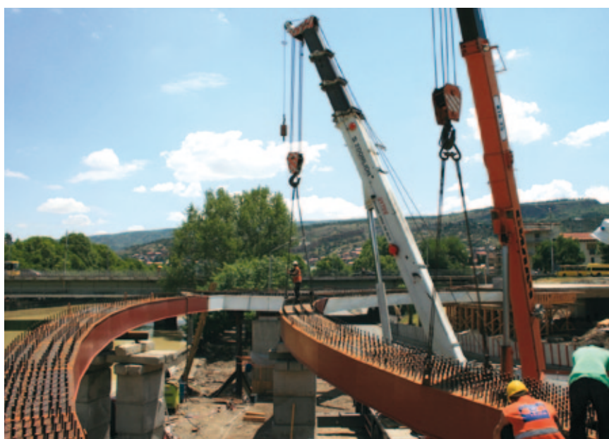
Fig.10, Laguna Bridge 01, lifting of steel girder
