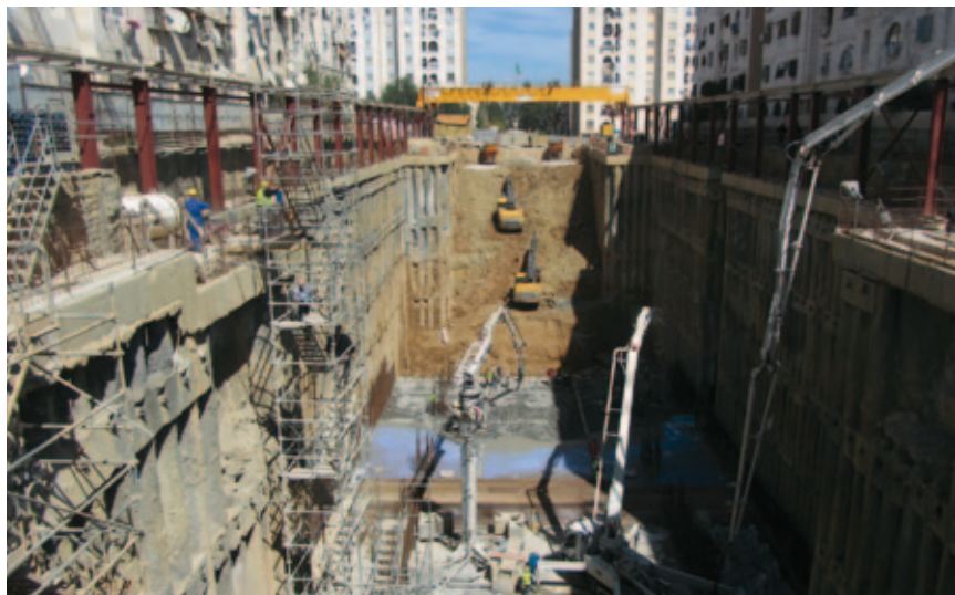
Fig. 13, Terminus Ain Naadja 2 area east, concreting of floor slab
