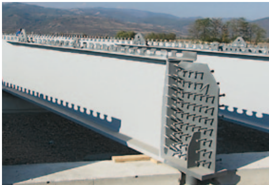
Fig. 12, Steel girder on site; double-line dowel bar in the bearing / framing corner area
