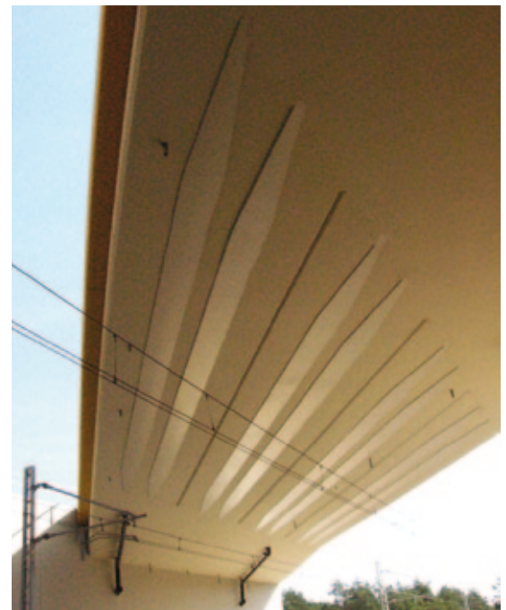
Fig. 7, Bridge WD-4, bottom view with external reinforcement adapted to the force flow
