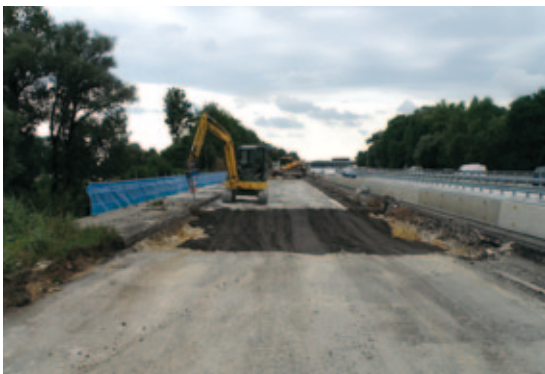
Fig.6, Demolition of caps and sealing
