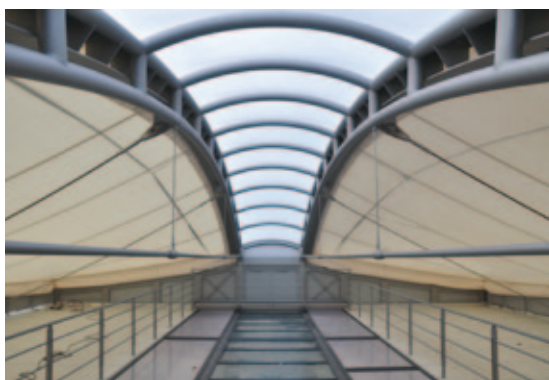
Fig.3, Intermediate roof structure with ETFE and PTFE membrane spans
